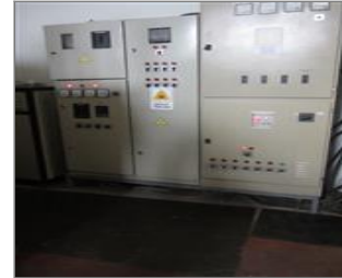
Photo of the inside of the main production hall Isolator mat.JPG
